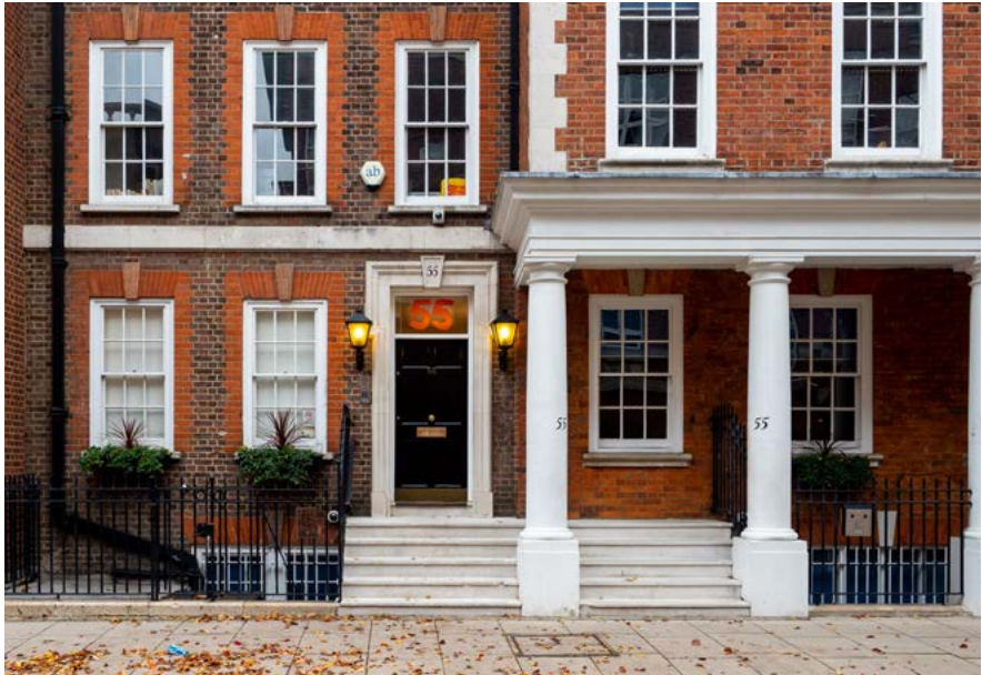
The main entrance to 55 Tufton Street, London, UK. A shared office space for a variety of lobbying organisations and think tanks. Photo R4vi from London, UK
